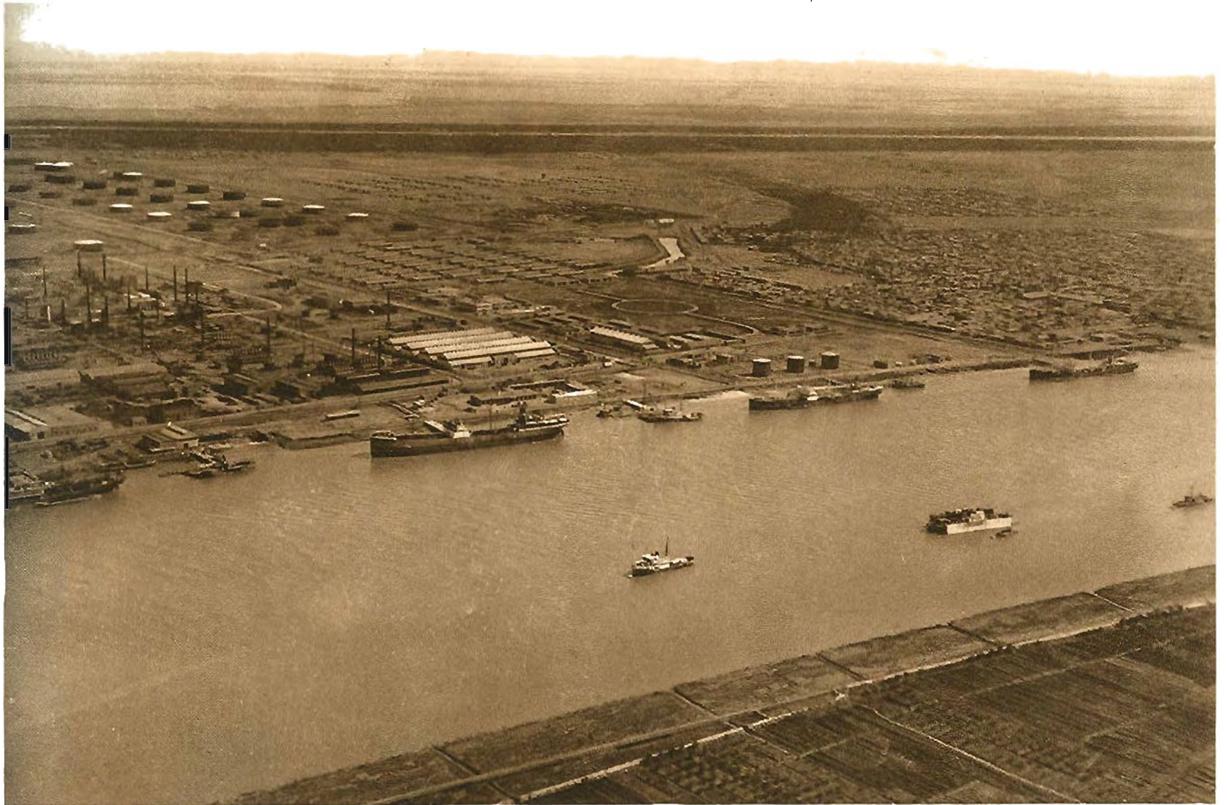
ABAOAN REFINERY, GENERAL VIEW, SOUTHERN SECTION
