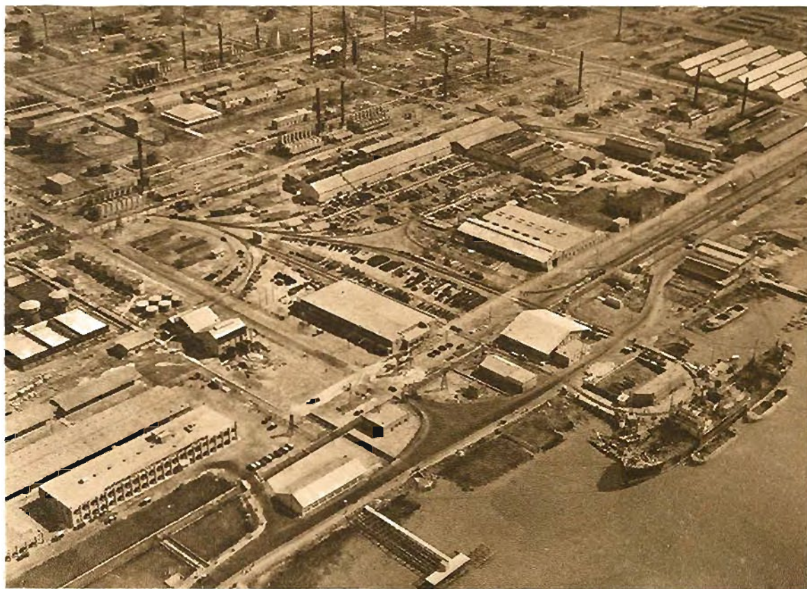
REFINERY, GENERAL OFFICES IN THE LEFT FOREGROUND
