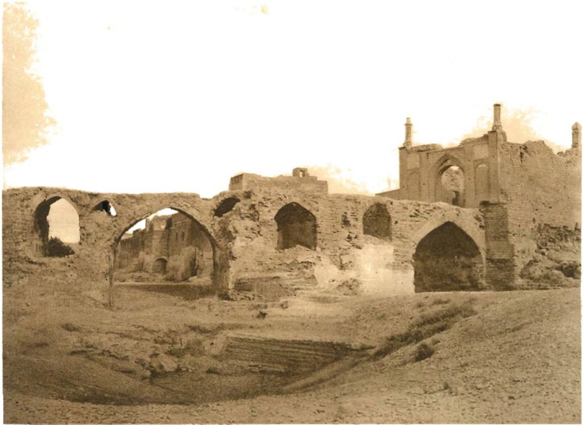
ENTRANCE TO VALERIAN BRIDGE
