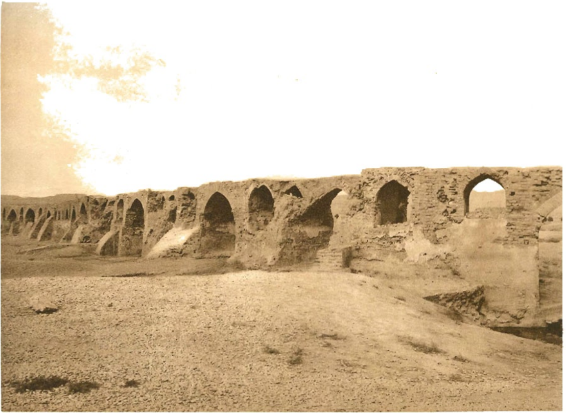
SHUSTAR RUINS OF VALERIAN BRIDGE
